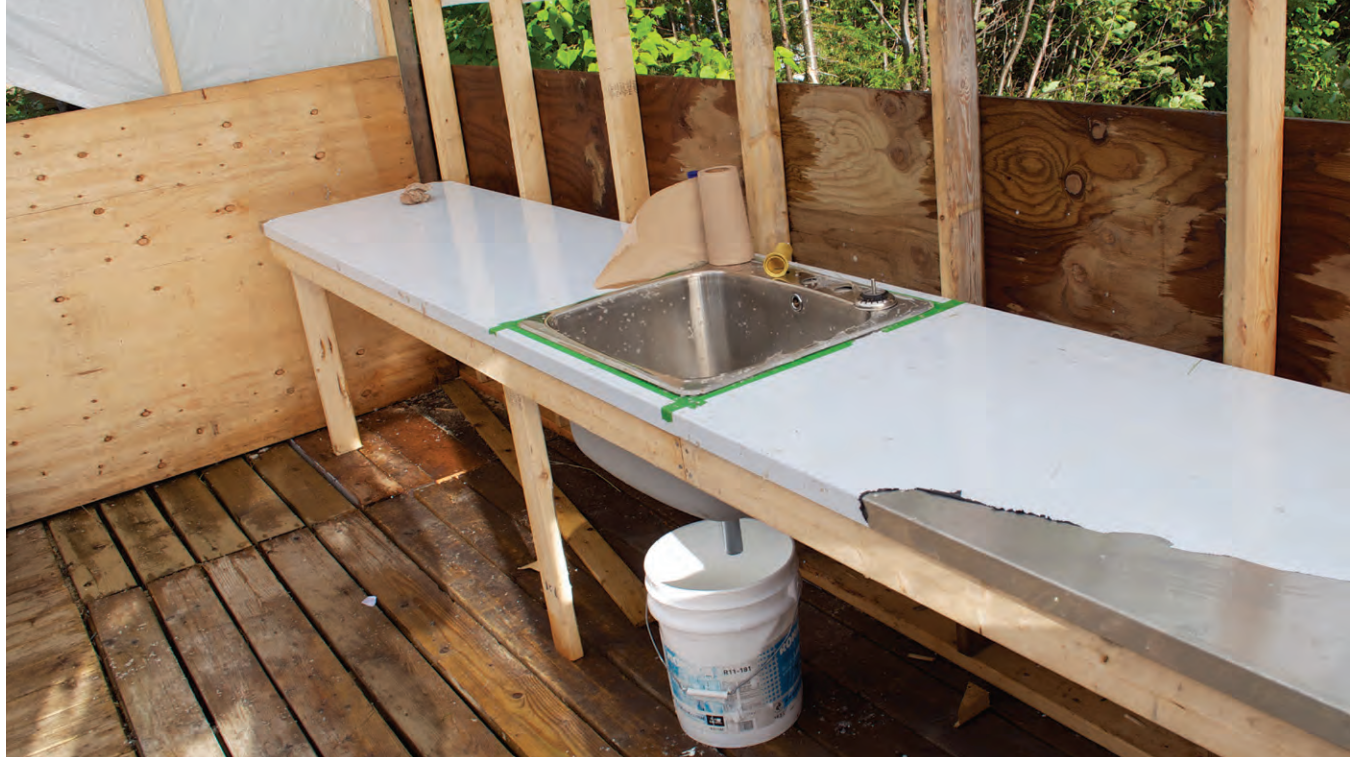
Newly installed stainless steel sink and countertop on the North shore
